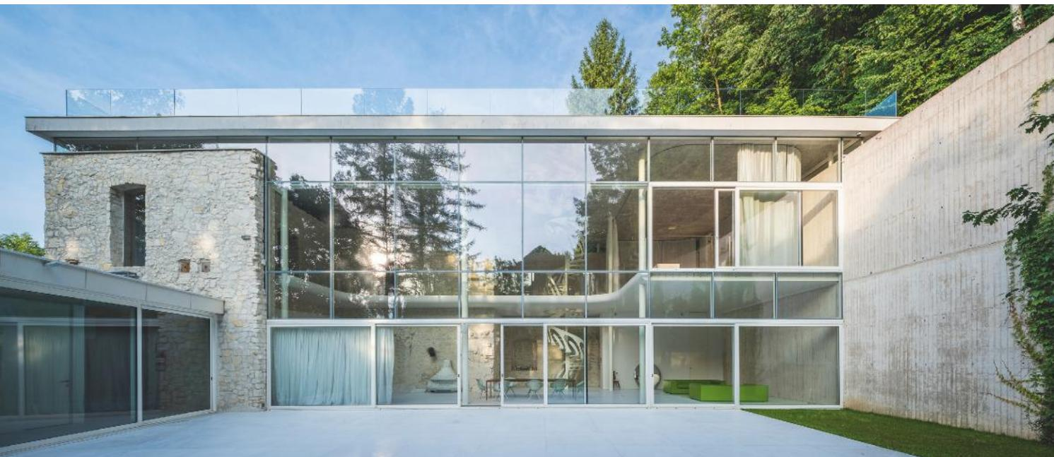
Above and below, a thin slab of pre-stressed concrete lifted on steel columns tops the main part of the project, which also features a west-facing floor-to-ceiling glass wall opening onto a generously planted courtyard with a small swimming pool
